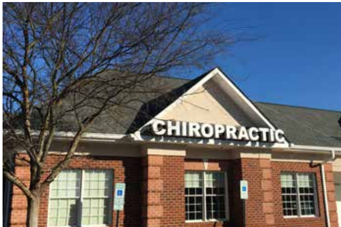
Gable and hip rooflines
